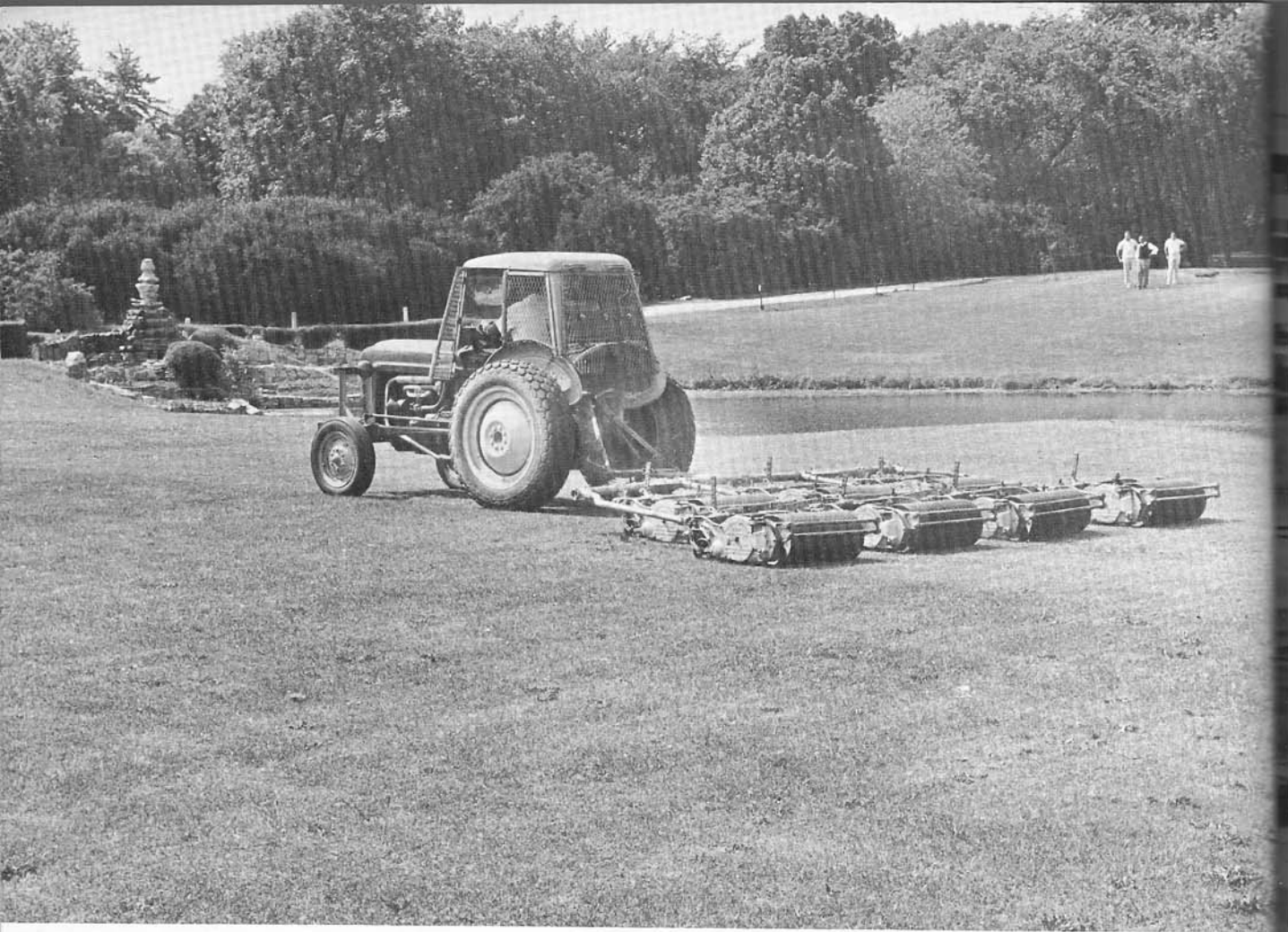
Waveland Golf Course, on Chicago's North Side lakefront, attracts over 70,000 players annually. Mowing and other maintenance is handled by this Ford tractor with seven-gang reel mower. Specially devised safety cage protects operator as he mows during play.
